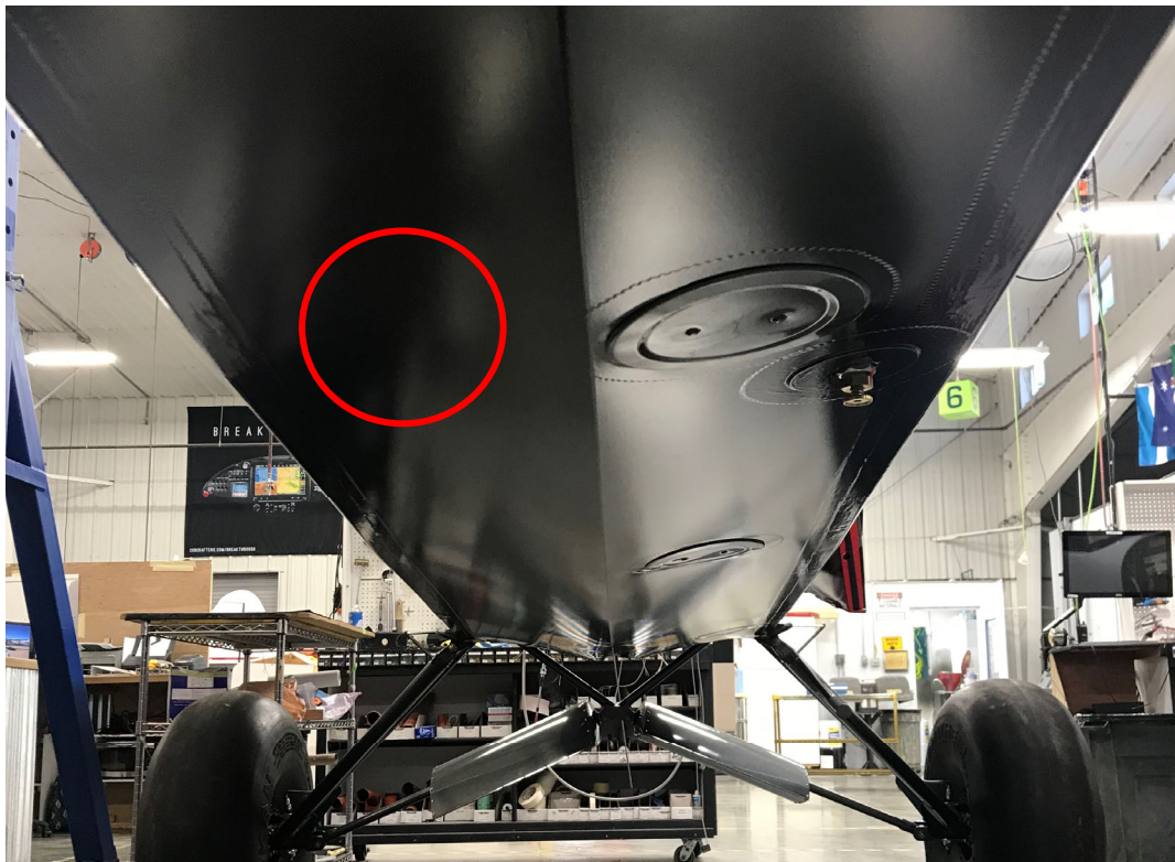
Figure 6 - New Inspection Panel Location
