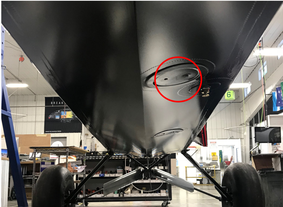
Figure 3 - Inspection Panel Location, Extended Baggage
