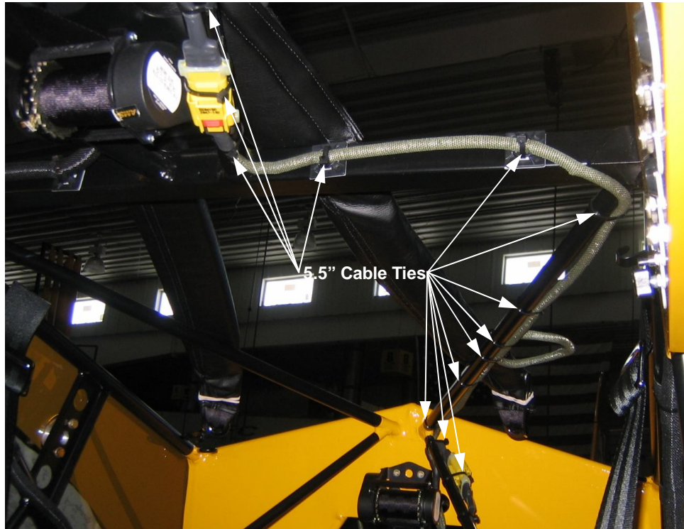
FIGURE 3 – Cable Tie Installation
