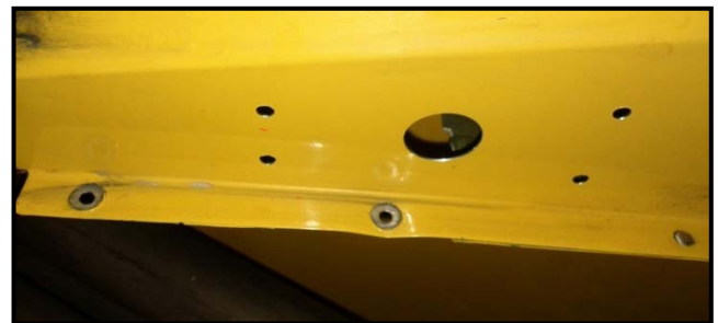
FIGURE 19 – Drilled Hole Locations
