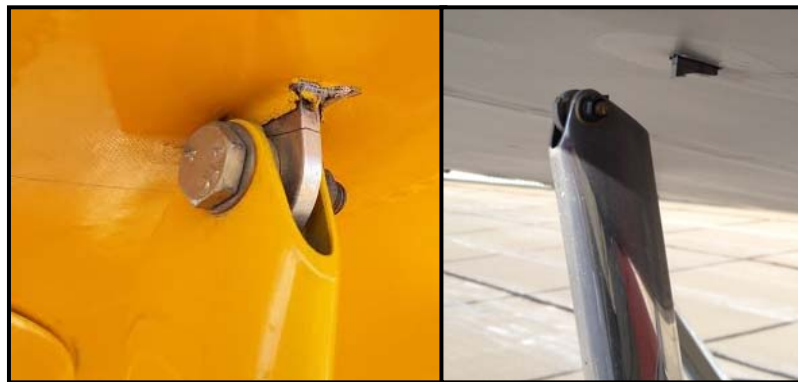
FIGURE 1 – Cracked and Sheared off Upper Bracket
