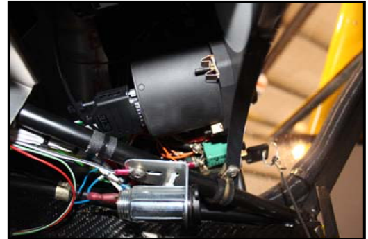
FIGURE 10 – Electronic Gauge as Installed
