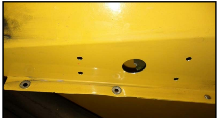
FIGURE 17 – Drilled Hole Locations
